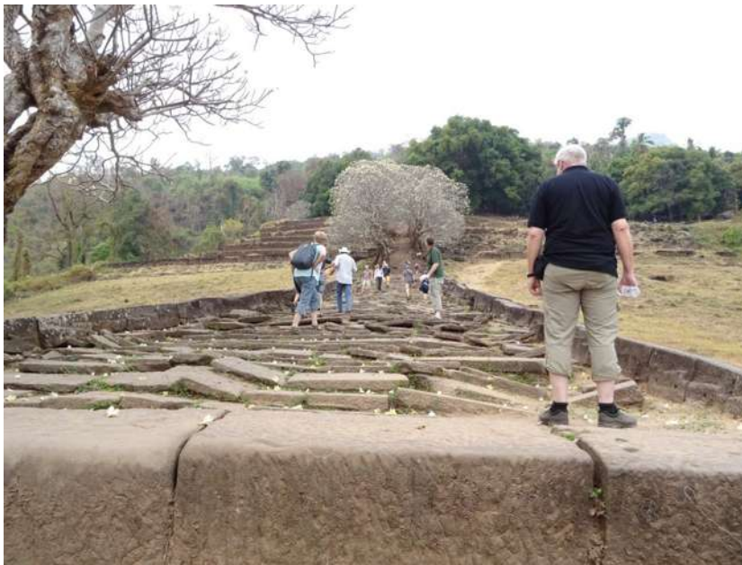
14. The central Vat Phou path surface, stairs and terraces would benefit from further consolidation (source: W. Logan).
